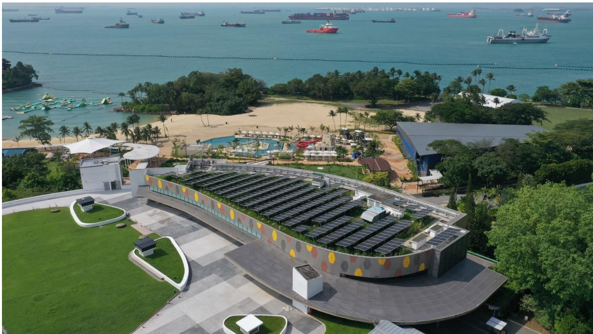
Solar panels installed on the roof top of Palawan Kidz City (Photo credit: Sentosa Development Corporation)
